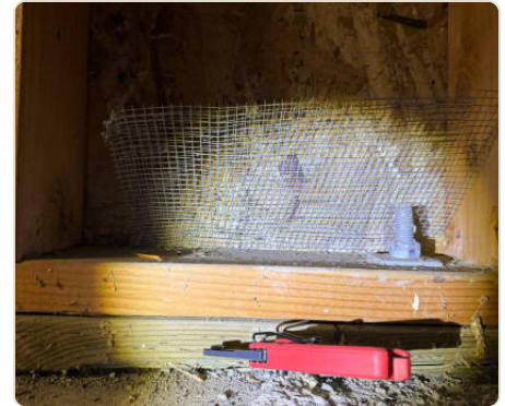
Plate 29. Screened foundation vent, mudsill, and an anchor bolt with nut and washer in place.
